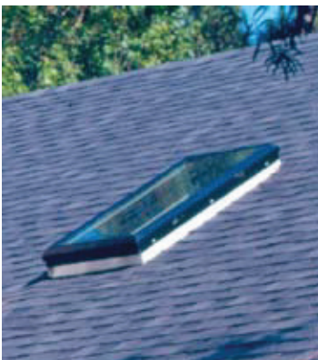
Use glass skylights; plastic will melt and allow embers into the home.
